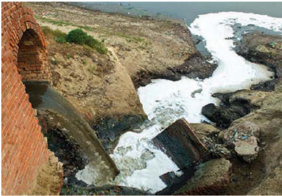
9.1 Discharge of polluted water in a water body
